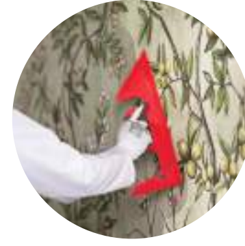
Remove the air from the center outwards and apply the wallpaper
