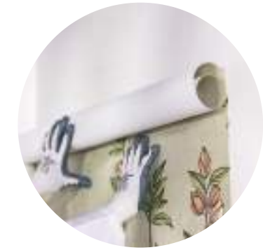
Lay the first panel checking for straightness
