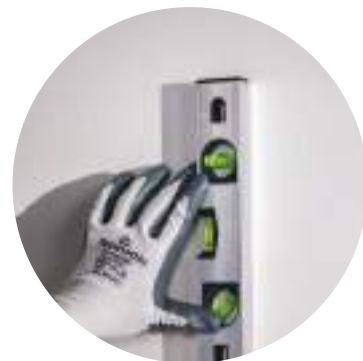
Check the straightness of the wall using a level indicator
